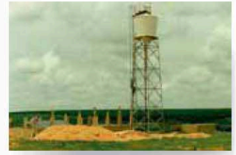
1991 - IVORY COAST PUMPING STATION
