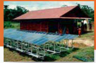
1991 - GUYANA FRANCE TELECOM SATELLITE STATION
